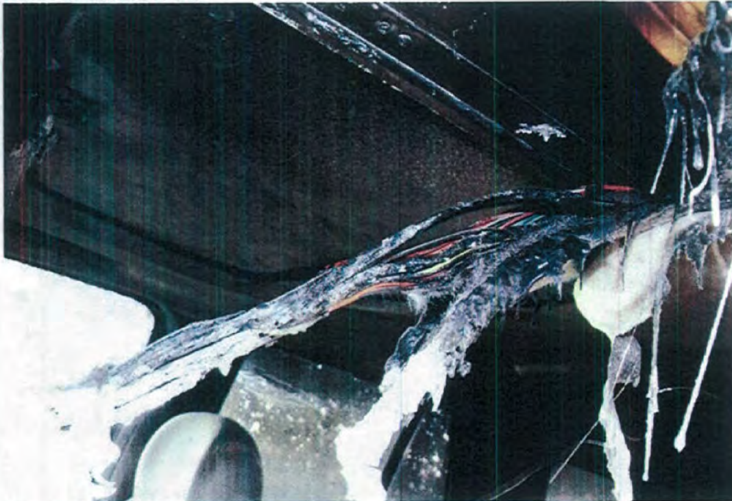
35. A view of wiring traveling along the headliner.
