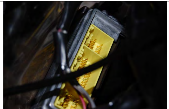
SRS ECU free from corrosion
