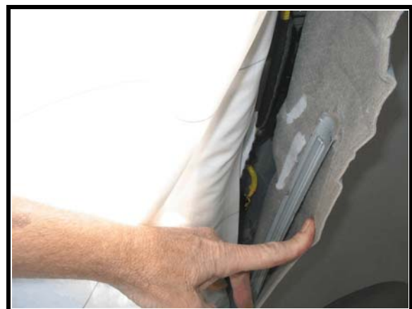
Figure 12. Aft aspect of metal stiffener (looking forward)
