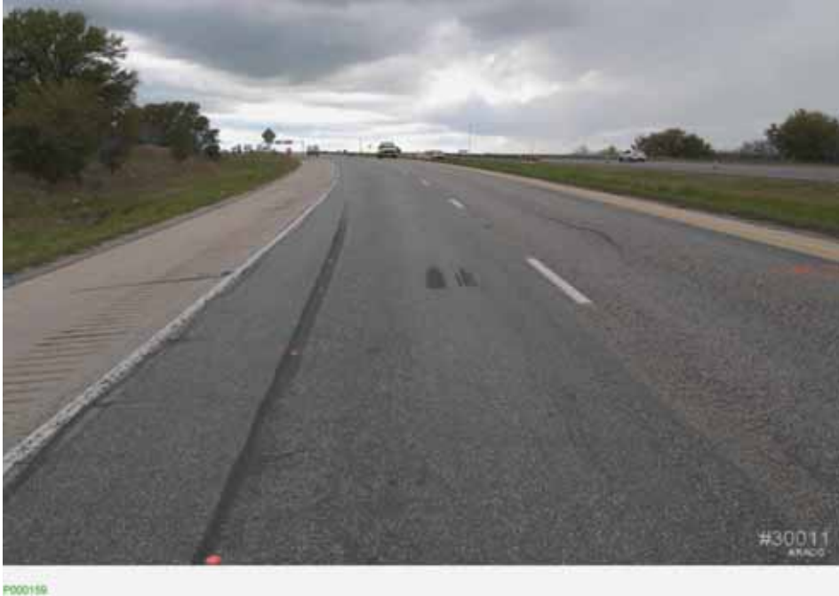
Figure 25- Northbound View Single Tire Marking
