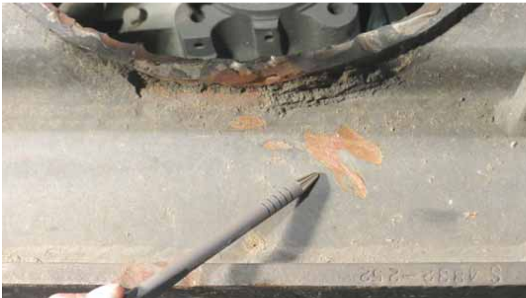
Figure 33- Americanos 60630 Driveshaft Escape Gouging Marks
