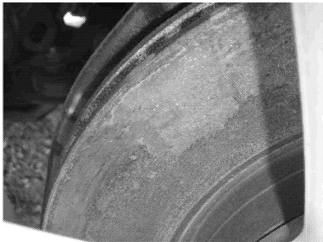
Photo 6: RHF rotor surface as viewed through the wheel aperture
