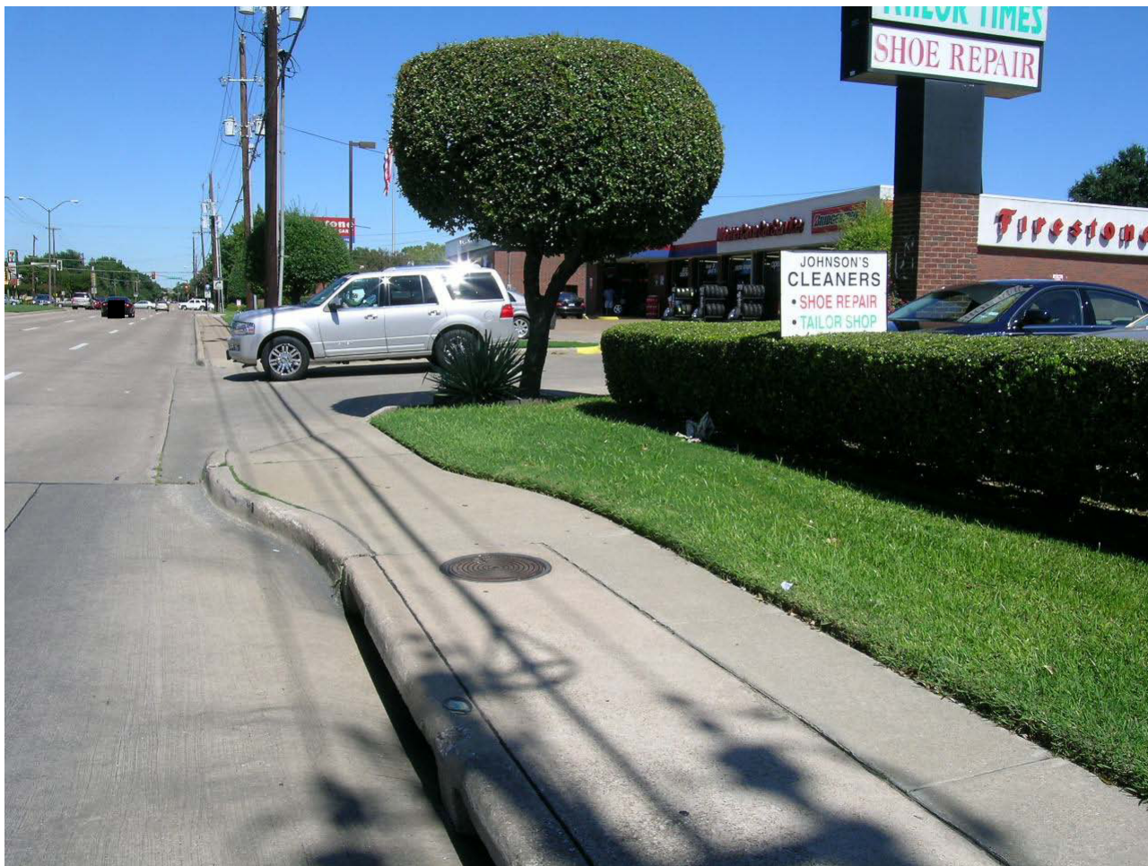
102. Closer view of the curb at the end of the storm drain with impact marks
