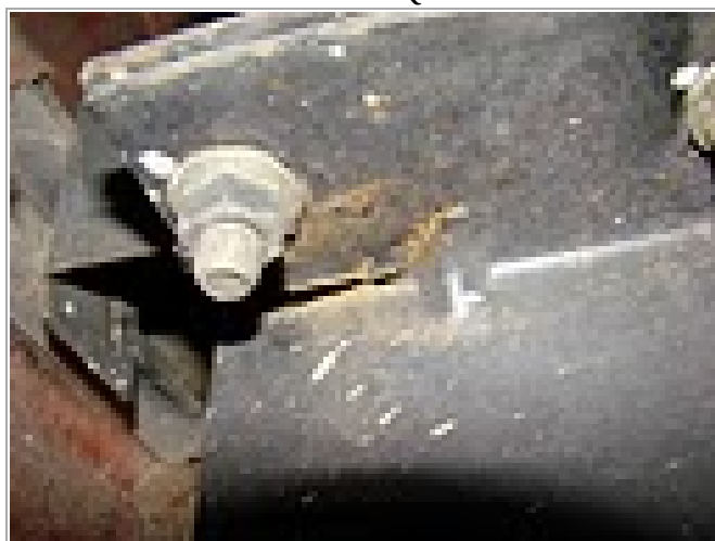
Photograph No. 4 – Cracked Attachment Bracket of Hitch Receiver Described in VOQ 10368002
