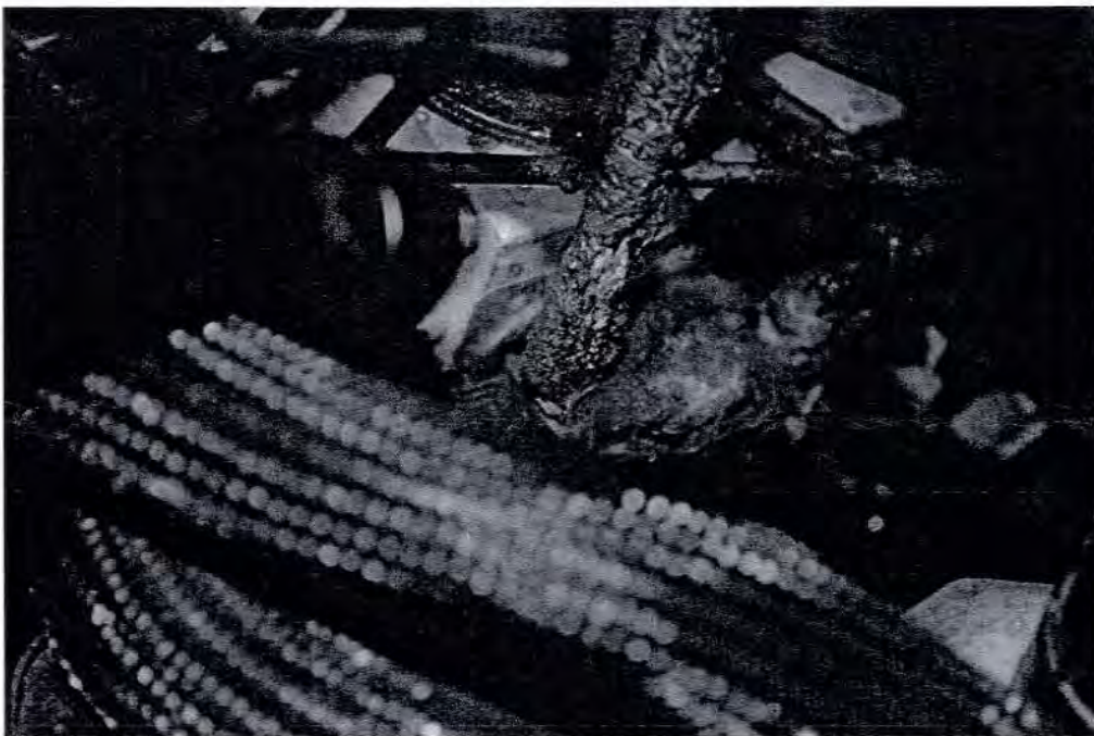
8. Wiring connected to brake control module is damaged from heat exposure originating from the module, not the result of wiring failure related to the fire cause.
