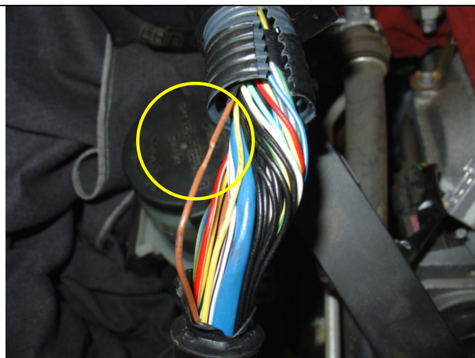
Broken wire seen here. Insulation is still intact.
