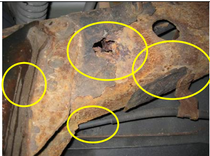
This is perforation found on drivers side above the rear leaf spring front mounting bracket
