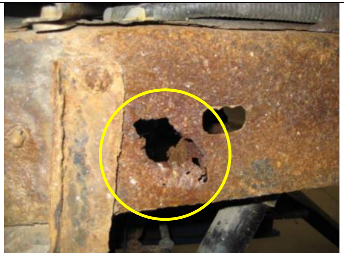
This photo is taken from the wheel well. Note the perforation through the metal.
