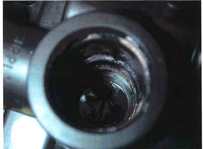
Double check valve bore – oil
