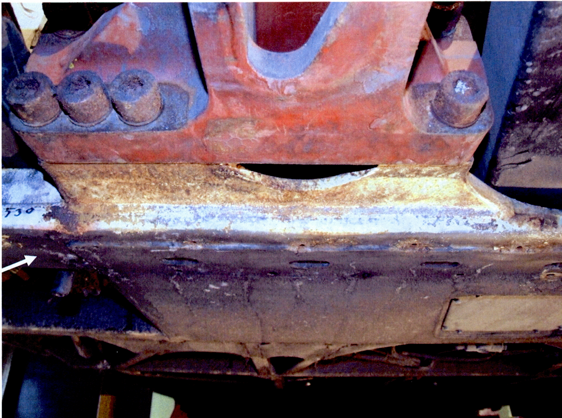
Figure 1 Hubner Joint Weld
