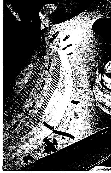
3.4" Crack @ 1,784K Miles Qty
