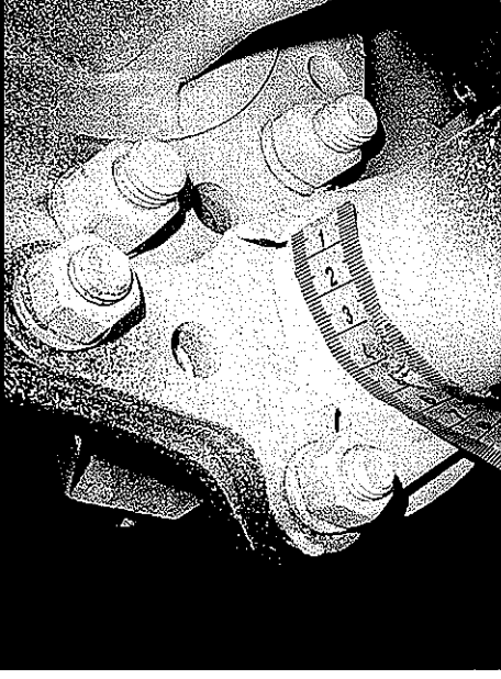
1.7" Crack @ 420K Miles
