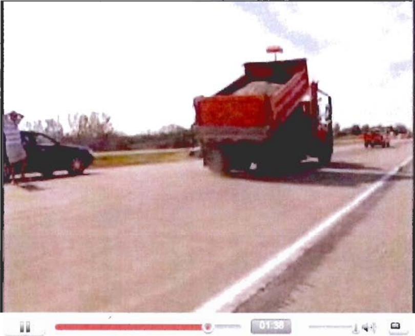
Figure 27 – The Iowa DOT Spread an Absorbent Material on the Roadway, Reportedly to Cleanup Split Diesel Fuel
