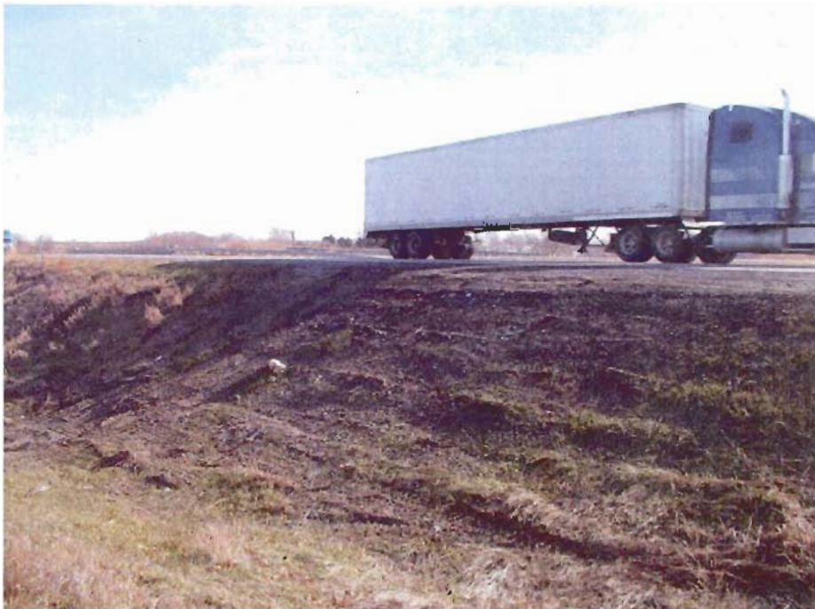
Figure 16 – View of the Right of Way Embankment at the Incident Site
