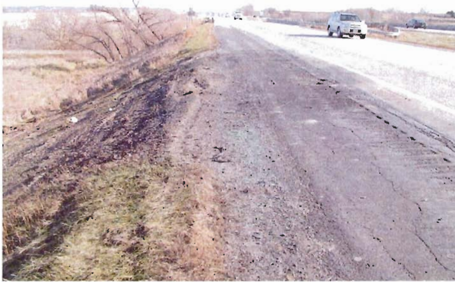
Figure 15 – Eastbound View of the Incident Site
