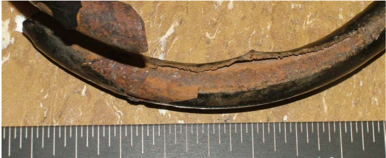
Figure 3 Cupping and Corrosion of Lower Coil
