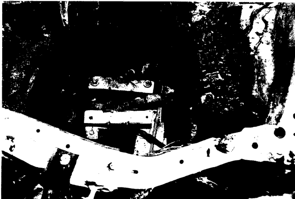
28. A view of the wiring beneath the battery tray intact.
