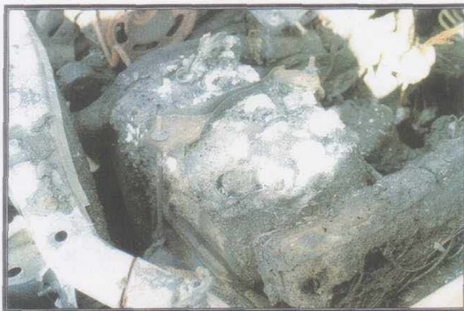
Photograph 9 (Heat damage to battery)
