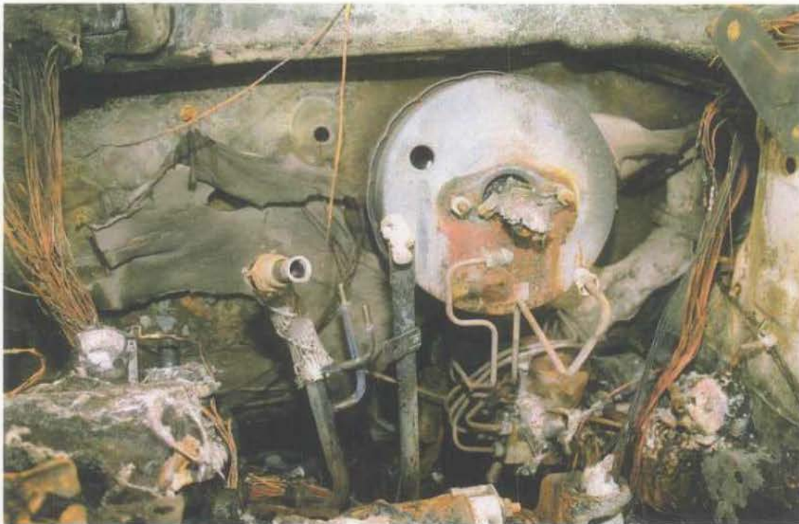
Photo No. 37: Overall view of the master cylinder and Injun block area.
