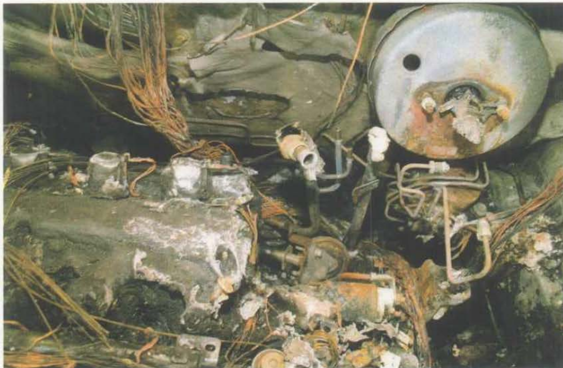
Photo No. 44: Overall view of the area of origin and engine block.
