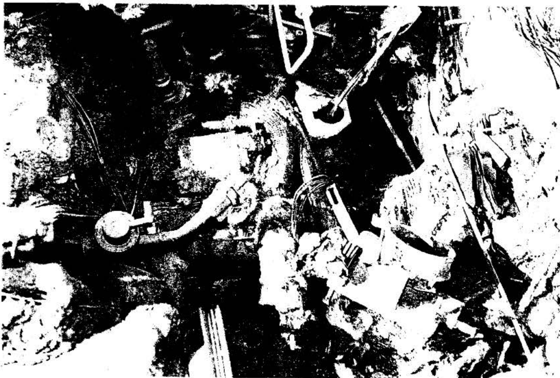
PHOTO #12: SURFACE DAMAGED HOSES AND CONNECTIONS
