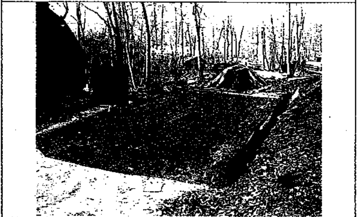
Photo 4: View of driveway following the removal of the asphalt and grading. Note the covered stockpile of excavated materials..
