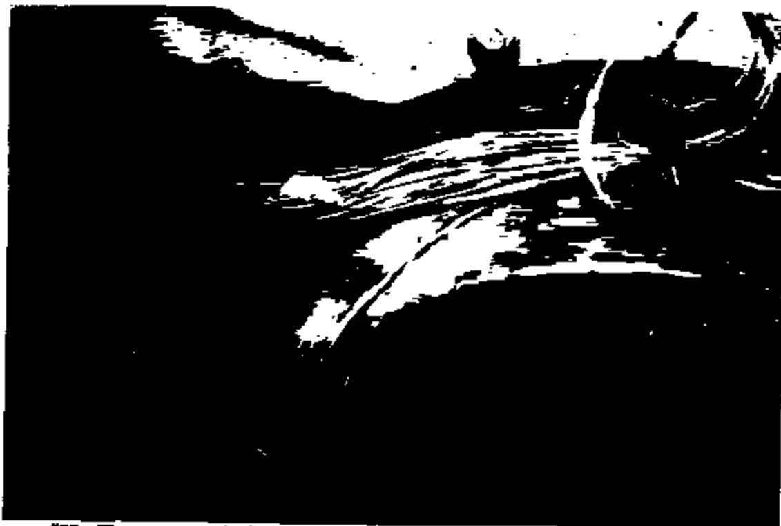
#39 - The vapor control valve wires were frayed, but they remained intact
