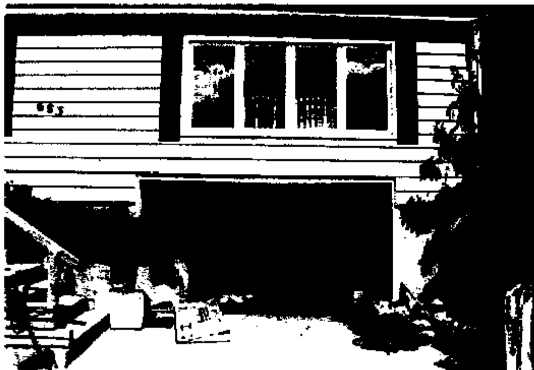
1. A view of the exterior front of the residence and garage.
