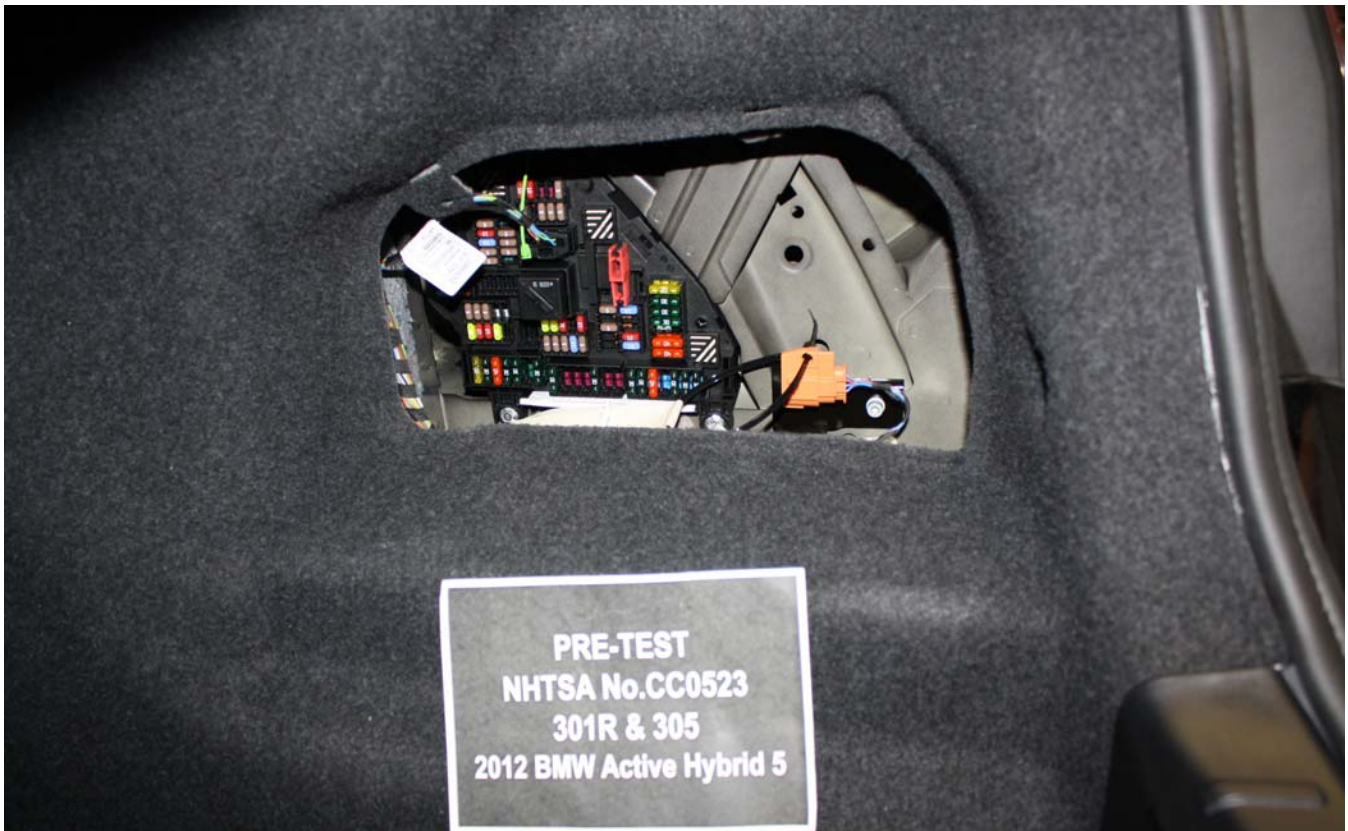
Figure A-48: Manual High Voltage Service Disconnect Removed (Location where removed)
