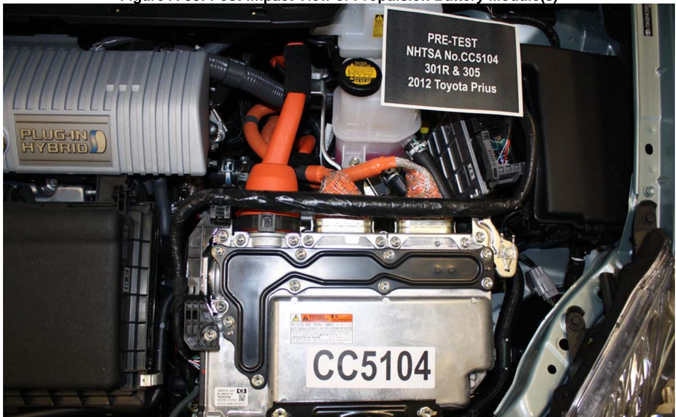
Figure A-56: Pre-Impact View of Electric Propulsion Drive
