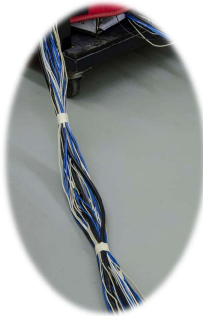
Figure 13-45. Final bundling of the "umbilical" cable
