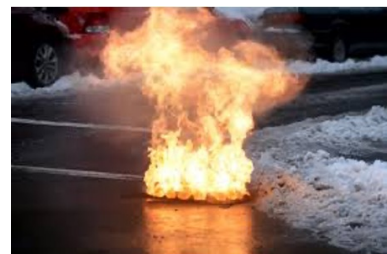
(i) Manhole fire
