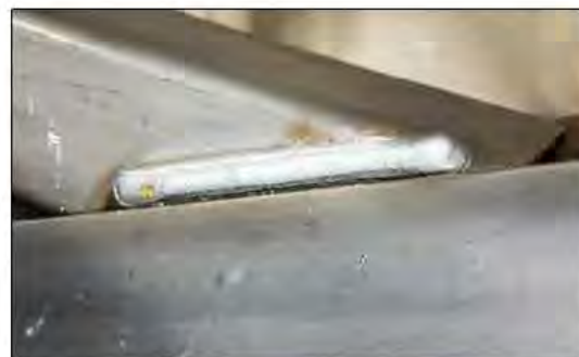
Figure 2 Weld missed one of the two pieces to be joined
