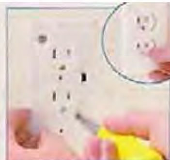
5. Push the device into the wall opening and mount it into the wall. Apply the wall plate.
