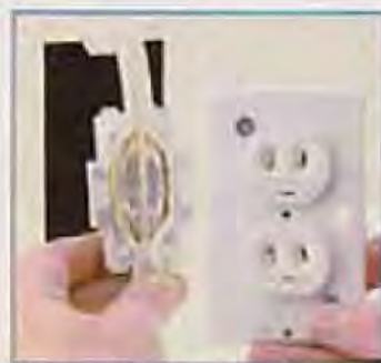
3. Load the slit Romex in the back of the device. No need to remove the insulation.
