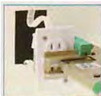
4. Snap close the front of the device onto the loaded back using the installation tool.
