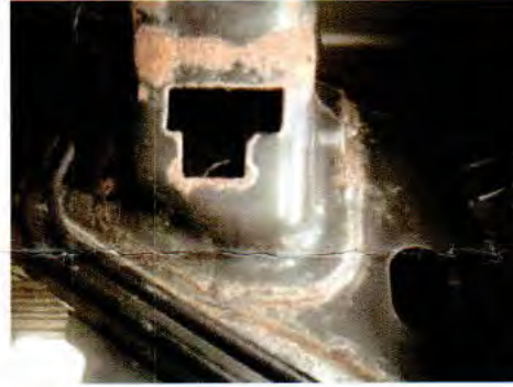
8/25/2016 E01 Comments: BACK MOUNTING PLATE IS JUST STARTING TO RUST ALSO.
