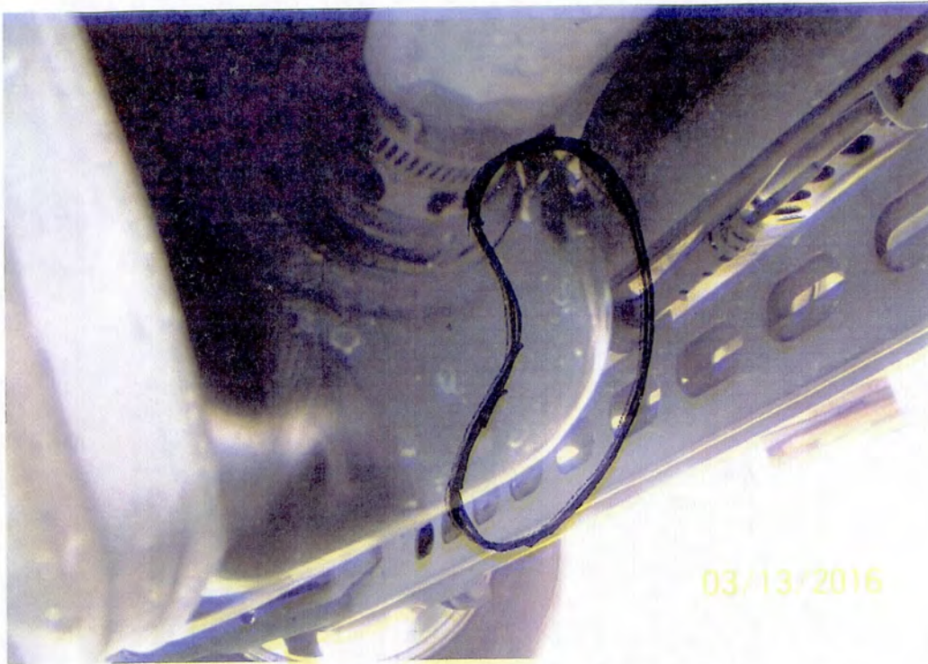
Gasoline leaks by the tank inlet
