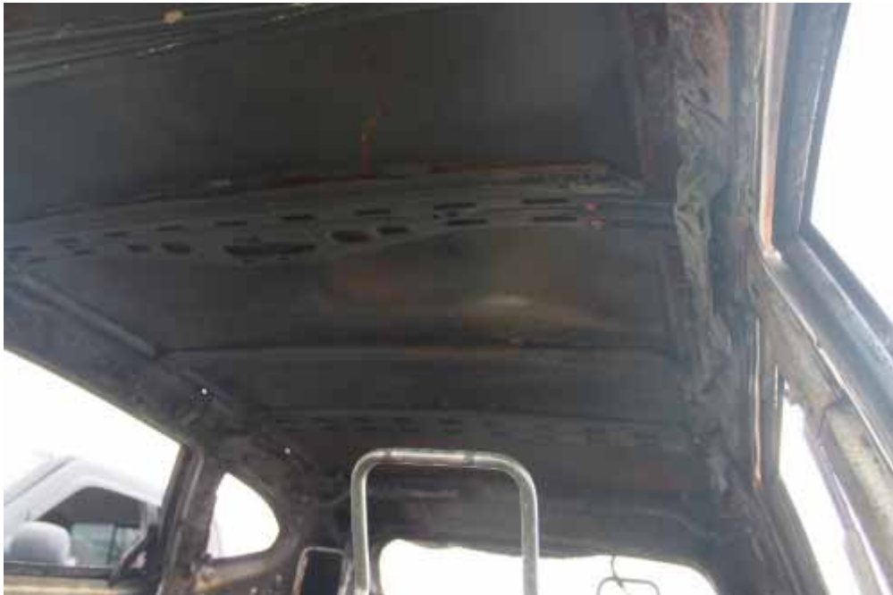
26. A view of the underside of the roof
