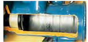
Grooves worn into the housing by hardened seals
