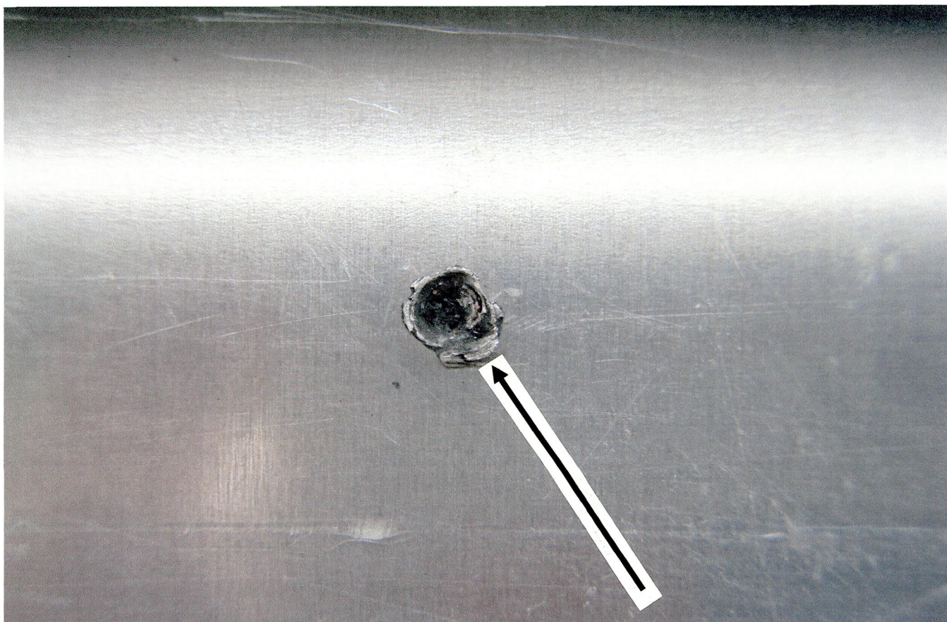
PICTURE 5 CLOSE-UP OF HOLE IN ALUMINUM TANK, LEFT SIDE OF FILLER NECK
